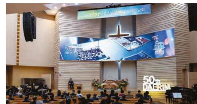
"As well as the main system, we also installed Outline's Vegas 24 enclosures, used as frontfill speakers and under-balcony delays to optimise coverage of the area of the congregation furthest from the altar," explains SungHwan Oh, Heksiba Multimedia's CEO. "In both cases, the Vegas 24 speakers were specified for their wide coverage pattern, ensuring maximum coverage from a small enclosure."
