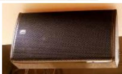
**Four ceiling suspended Outline Vegas 12 speakers provide the main sound reinforcement in QBC's sanctuary**
